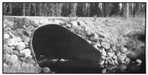
Washed out culvert replaced with a new arched culvert having sufficient opening.
